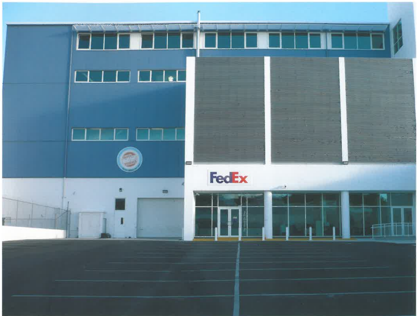
New Venture House's parking lot accommodates 60 cars and 60 bikes making it convenient for retail and office tenants, as well as those using the self storage units
